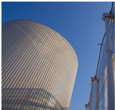
04/ Heat/cold storage tanks
